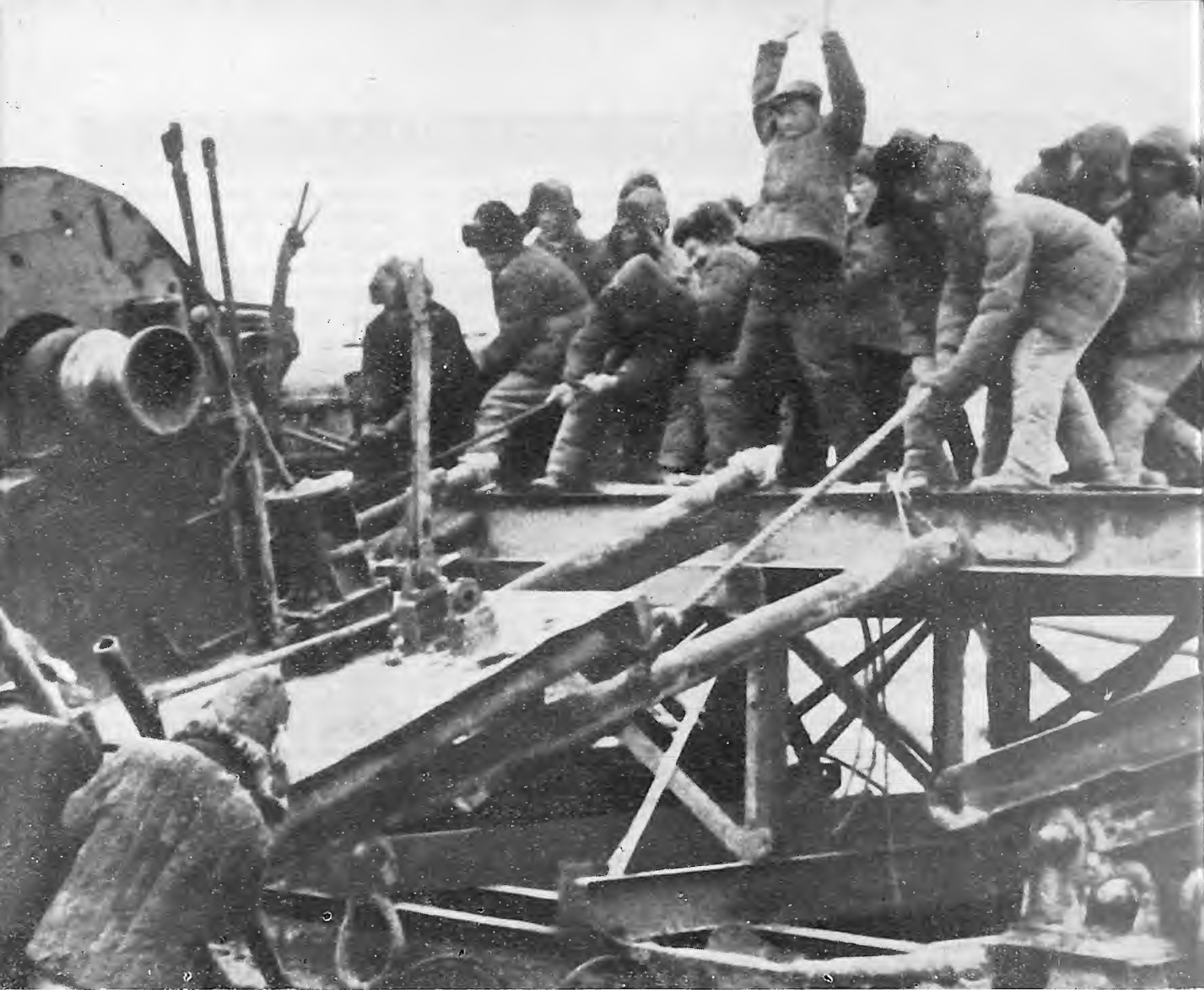
When cranes had not arrived, Drill Team No. 1205 led by Wang Chin-hsi moved drilling equipment with shoulders and crowbars.
